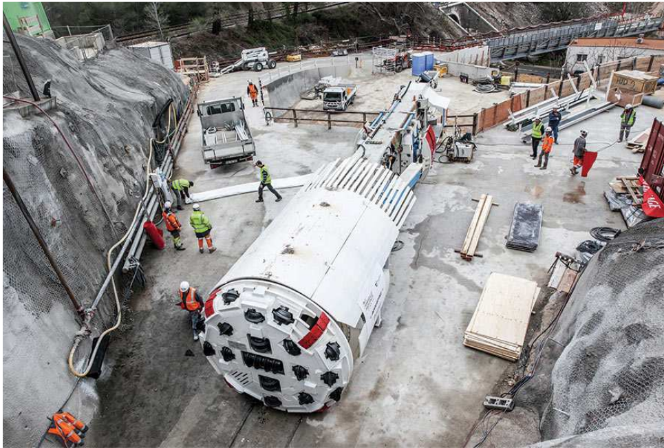
The TBM used during the excavations
