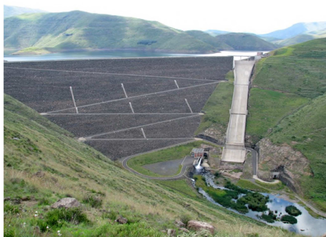
The Itare Dam next to Nakuru City for the new water supply system © Alpina Archive
