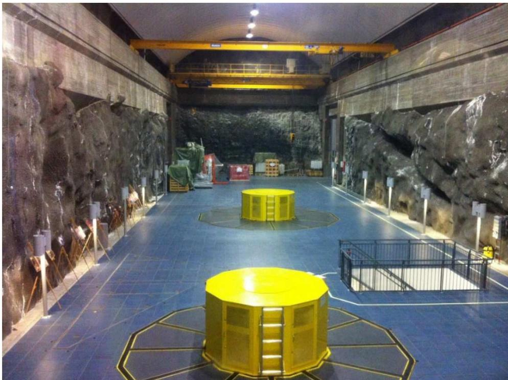
Fig. 2. Example of design of recent Norwegian powerhouse cavern with exposed rock at end walls and thin layer of sprayed concrete combined with spot bolting at the sidewalls.
