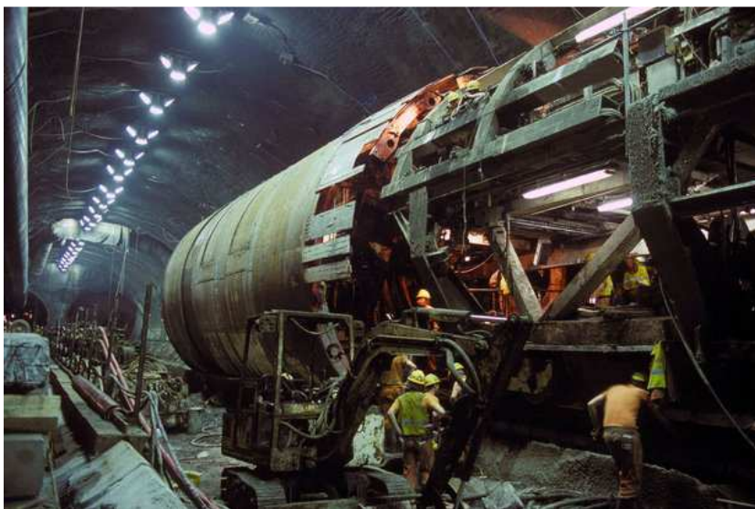
Underground construction site
