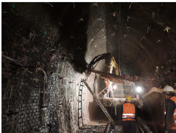
Strengthening of Bricchetto railway tunnel © www.impresaluiginotari.com
