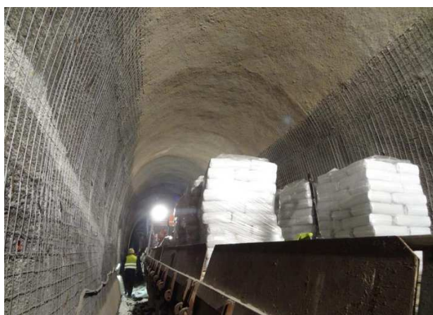
Fire protection works in Fey tunnel © www.utt.mapei.com
